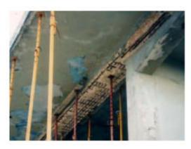
**MAXRITE**® **500** the applicator can place in about 10 minutes, because after this time, the mortar will have started its setting and will no longer be workable.
